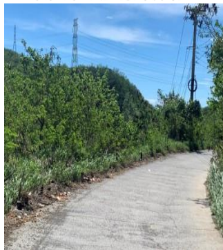
(前方)防撞護欄損壞
